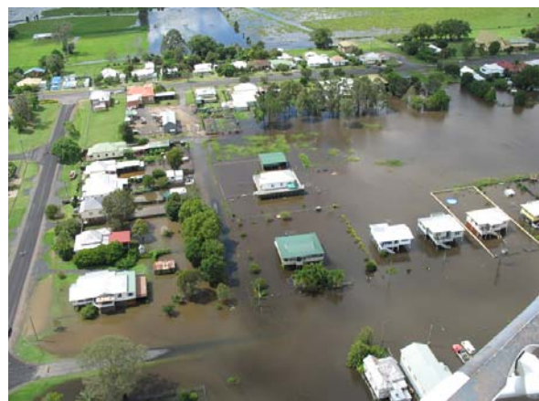
Flooding from the Richmond River at Coraki, January 2008
