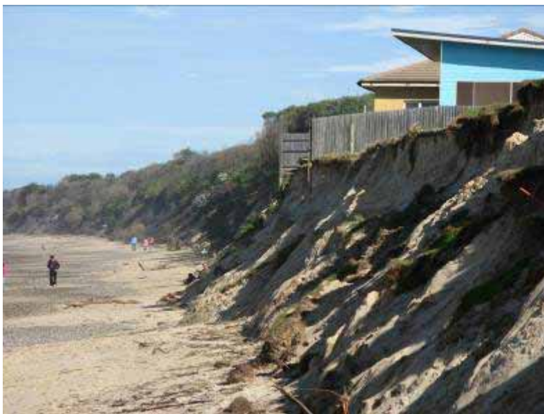
Coastal erosion at Old Bar
