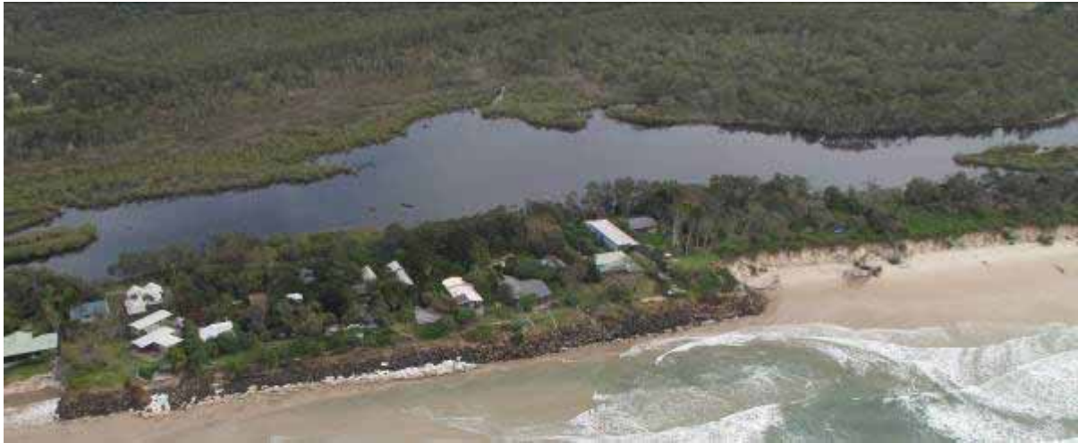
Seawalls and coastal erosion at Belongil Beach, Byron Bay
