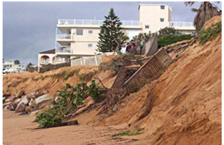
Erosion at Collaroy
