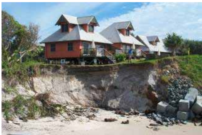
Coastal erosion at Belongil Beach, Byron Bay
